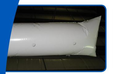
Polyducts are a low cost, yet highly efficient way of distributing and mixing conditioned air. They are designed to diffuse and provide ventilation evenly over large areas.
